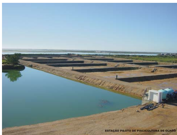
Figure 3.9 – Earthen ponds in the Ria Formosa lagoon (IPIMAR – National Institute for Sea Research-experimental station).
